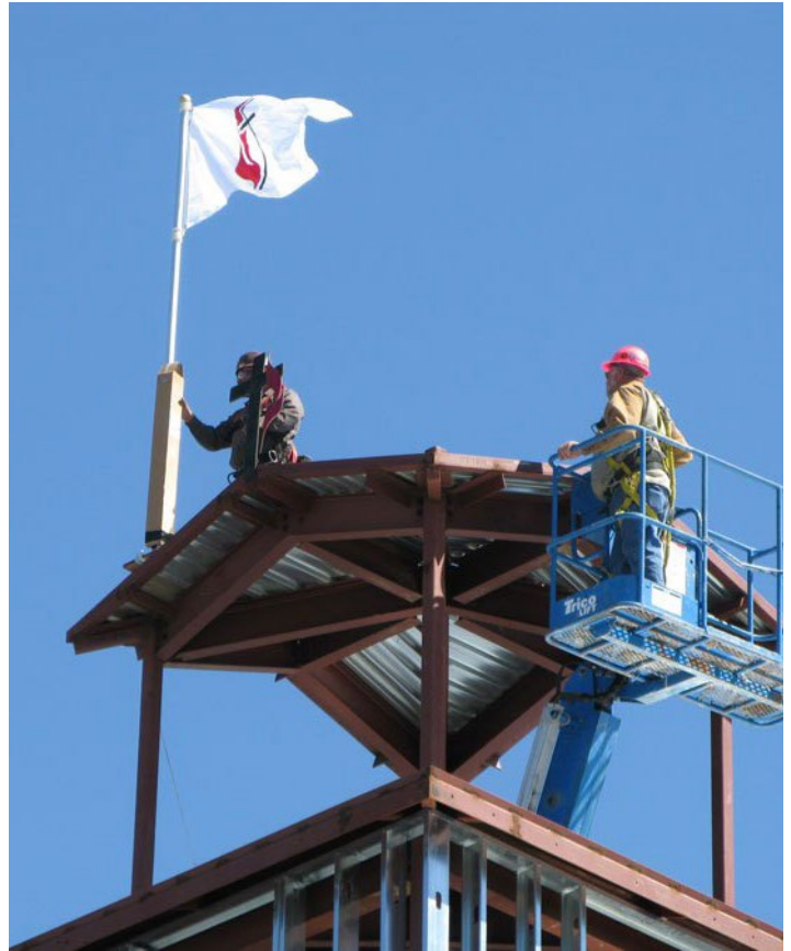
FUMC Dickinson Topping-Out
