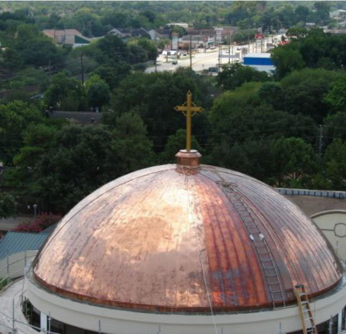
Christ the Redeemer Catholic Church Under Construction
