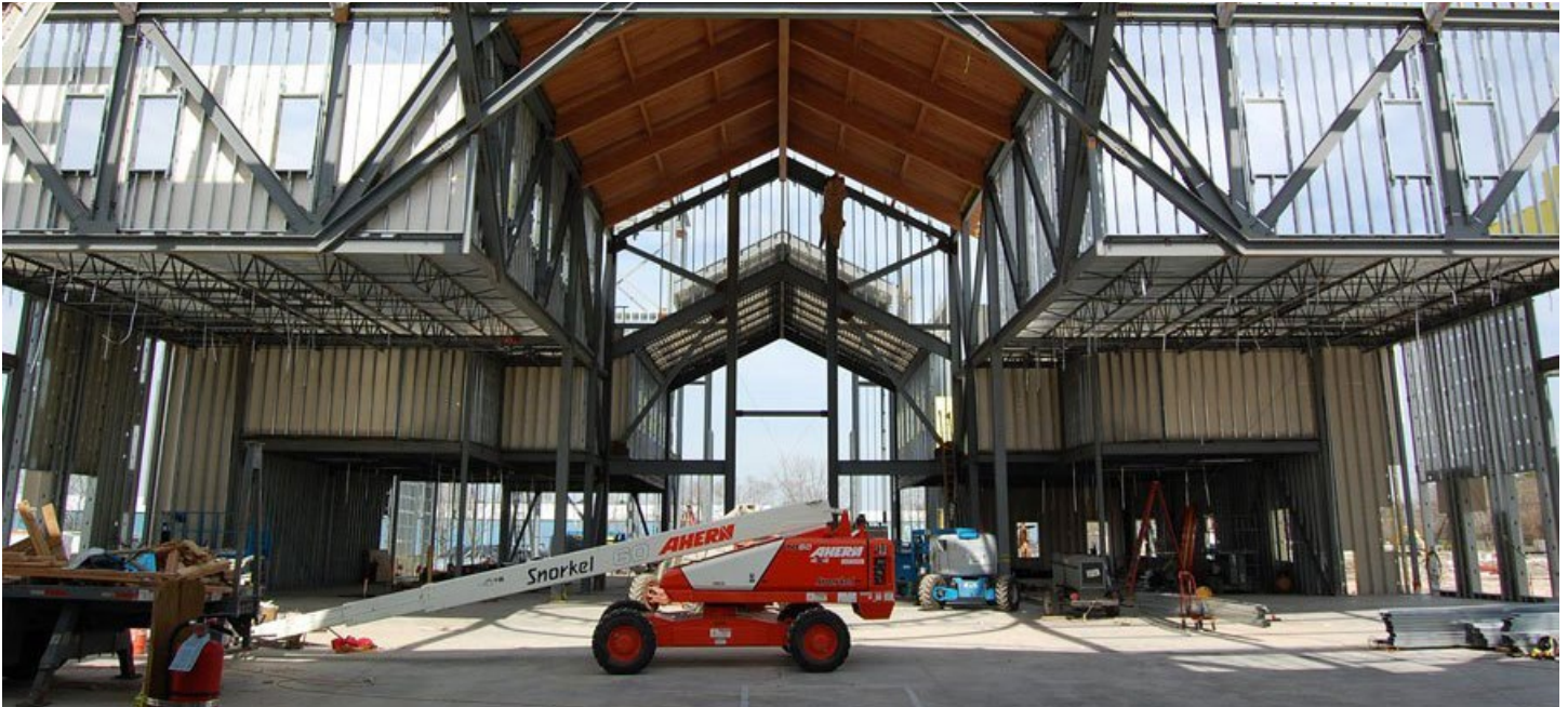
Catholic Church Under Construction
