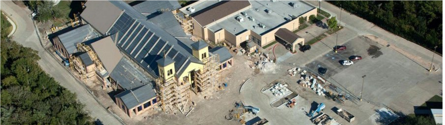
Mary Queen Catholic Church Friendswood Under Construction
